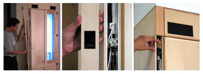
Figure 8. PlaceLab interior testing one aspect of Open Source Building: Integrated Interior Infill (I3) components with sensing and addressable lighting infrastructure. Shown are hinged, accessible sensor bus raceways. All cabinets use the same embedded connections and technologies, simplifying installation and increasing flexibility. The facility contains hundreds of modular sensors.
